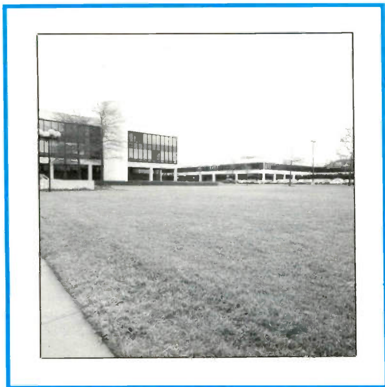
From headquarters in Secaucus, NJ, Matsushita Services Company (MSC) coordinates a U.S. network of factory servicenters, independent servicenters, self-servicing dealers, parts and accessory stocks and training sessions.
