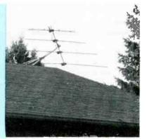
This tripod roof mount and rotor survived a windstorm safely, but the antenna suffered bent elements and a broken 300  $\Omega$  twin lead.
