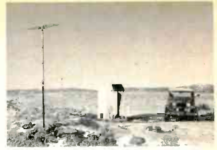
Two masts with antennas, a panel of solar cells, and an old refrigerator cabinet—but no power lines—make up the one-channel translator on Johnny Moore Mountain.
