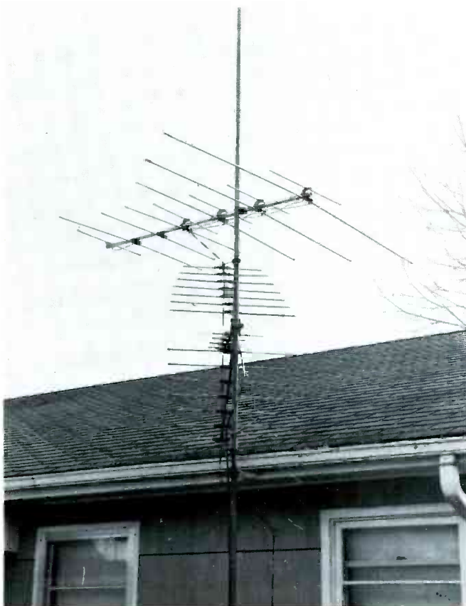
Separate UHF and VHF antennas at your editor's home were used to compare signal quality with a new cable installation.
