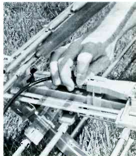
Fig. 3 When coax cable is used with a 300-ohm antenna, install a good-quality weatherproof matching transformer at the antenna.
