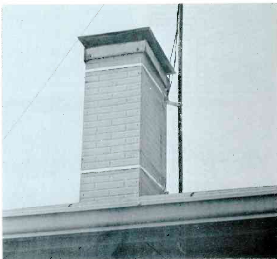
Fig. 8 Chimney mounts are favored by many installers. Place the straps as far apart as possible.
