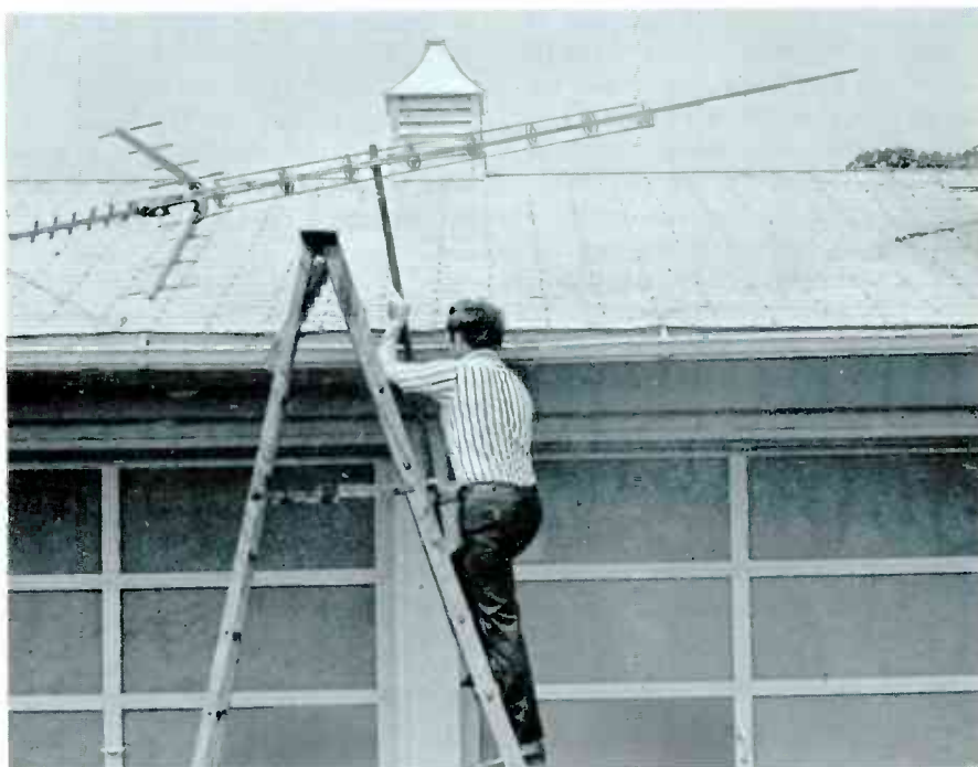
Fig. 7 Carry the completed antenna/mast assembly up to the roof. Don't attempt to assemble it on the roof.
