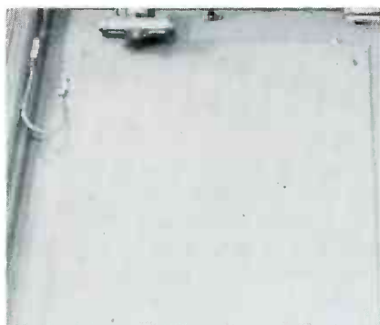
Fig. 7 Plywood or pressed wood should be installed over the wires on a door to protect against damage to the wires.
