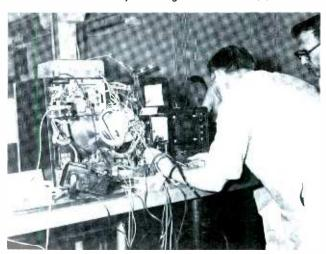
When troubles got tougher there was no hesitation in using a color-bar generator and scope to isolate the defect.
