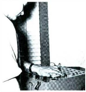
6. The lesson had been learned to test tubes first, or in case of transistors to check for change in collector volts while intermittently shorting base to emitter.
