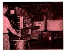
Engineer uses resolution and registration charts to adjust color-TV camera.
