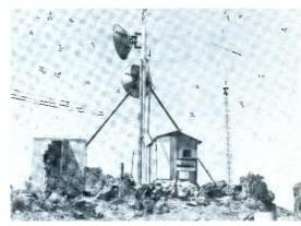
Two transmitting antennas, facing in slightly different directions, broaden coverage pattern of this UHF translator.
