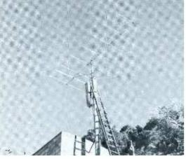
Compact installation has UHF transmitting antennas (in weatherproof housing) mounted on same mast as VHF receiving antenna. Note concrete-black shelter.
