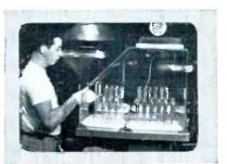
Guns await final assembly in this pressurized plastic housing. Blower at top maintains pressure, prevents dust from entering nousing.
