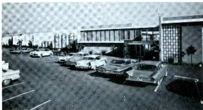
Whittier, California — The Casa Linda, located in a strong signal area, has two Wizard systems of 44 outlets each with: excellent reception and no amplification.
