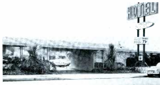
Los Angeles, California — The Skyway's Hotel has a Wizard system for each individual unit. Each system provides from 10 to 24 outlets without amplification.
