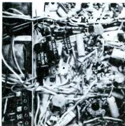
Fig. 4. Appearance of the Olympic vertical circuit when brought to the shop.
