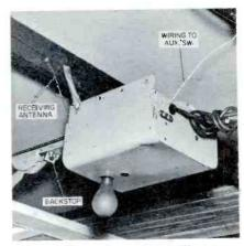
Perma-Power Operator Installation
