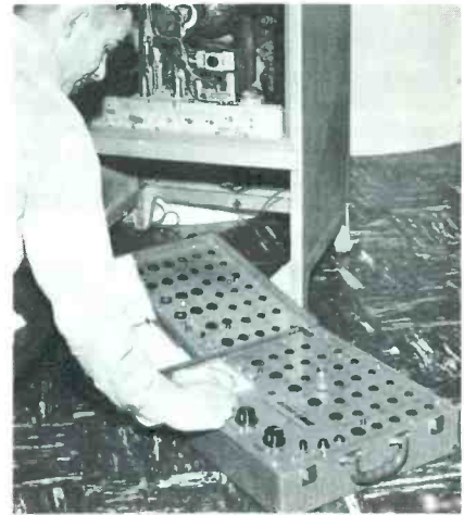
Fig. 9. "The Dyna-Quik" Tube and Transistor Tester features pre-wired sockets.
