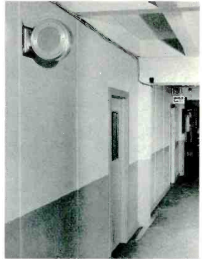
Fig. 2. Bi-directional speaker for paging service in long hallway.
