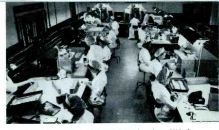
Separate facilities are maintained for the exclusive processing and manufacture of high reliability capacitors. Only specially trained, highly skilled operators, who wear special clothing to prevent any possible source contamination, work here.
