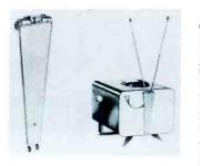
The "Tuk-A-Tenna," designed by JFD Mfg. Co., Inc., 6101 16th Ave., Brooklyn, N.Y., is a "rabbit-ears" indoor antenna that collapses out of sight behind the TV set when not in use. The base of the antenna is fastened to the back of the receiver. An optional feature is an
