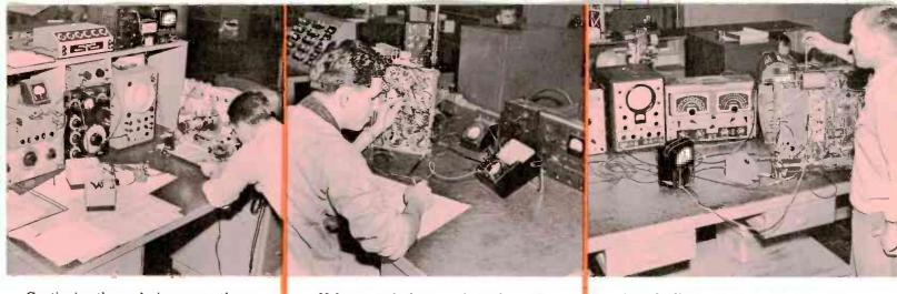
Continuing the analysis process, the receiver progresses through 13 separate operations: Data is gathered and recorded on controls, resistors, RF and IF components, transformers, chokes, speakers, deflection components, tubes and other parts.
