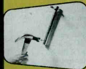
Nail up mounting bracket.
