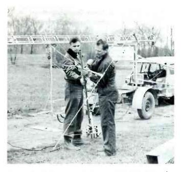
Fig. 5. Installing Antennas and Harness on Mast Assembly. 📥
