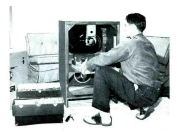
Fig. 6. Preparing to Replace a Cabinet-Mounted Picture Tube,
