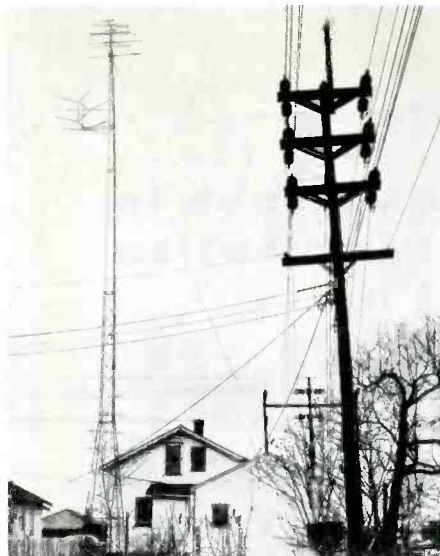
Fig. 14. A High Tower Close to Power Lines Can Cause Trouble. (Courtesy NFPA.)
