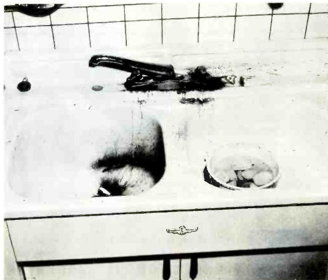
Fig. 16. Sink Where Stray Currents Entered Via Sewer Pipes to Water Pipes. (Courtesy NFPA.)
