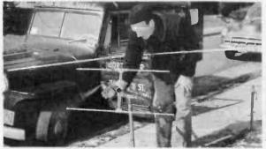
Edward Weigand, Farr service man. sprays Krylon on ertire antenna. Krylon shuts out moisture, rain, salt spray—prevents corrosion and pitting—keeps picture quality at peak.
