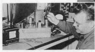
1. ISOLATING THE TROUBLE—Plug the power cord of the chassis into LOADCHEK and note the reading. With your eye on the large meter remove the rectifier tube and you can tell immediately which side of the tube the trouble is on. You have already eliminated 50% of your probing time.
