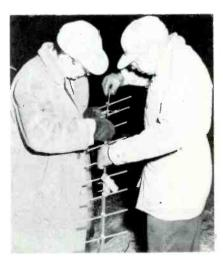
Figure 16. Photograph of the 12-Element Yagi being Prepared for Installation on the Tower.
