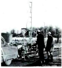
Figure 4. Installing Tubular Leadin for Testing Purposes.
