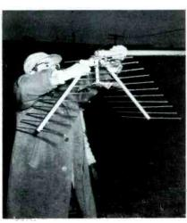
Figure 10. The Corner Reflector Being Mounted on the Mast in Preparation for its Test.
