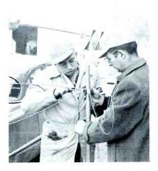
Figure 6. The Clover V-Beam (Telrex, Model 100) Being Installed on a Section of Mast.
