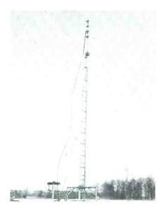
Figure 1. Portable Antenna Tower Showing Rotator Used for Orientation of Antenna.
