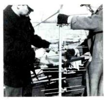
Figure 18. Photograph Showing the Colinear Antenna Being Attached to a Section of Mast.
