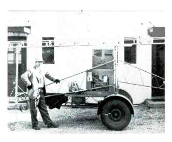
Figure 16. Trailer-Tower Loaded with two TV Receivers.
