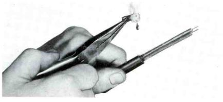
Figure 6. Sealing the Anaconda ATV-270 Line.
