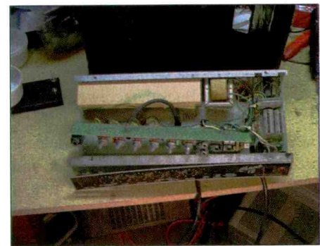
Figure 8. The main circuit board removed. Every nut on every control and jack had to be removed to get this far. Also, what looks like a cardboard box is the reverb unit.
