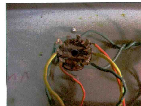
Figure 10. A lot of hand wiring and soldering go into most tube amps.
