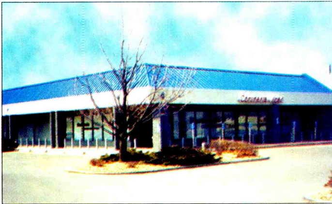
Figure 5. The signage on the building is minimal, but the neat appearance and the list of products sold in the windows attest to the potential customer this is a well managed operation.
