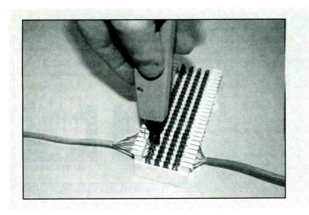
Figure 4. A 66 block. This type of connecting block is most often used for telco.
