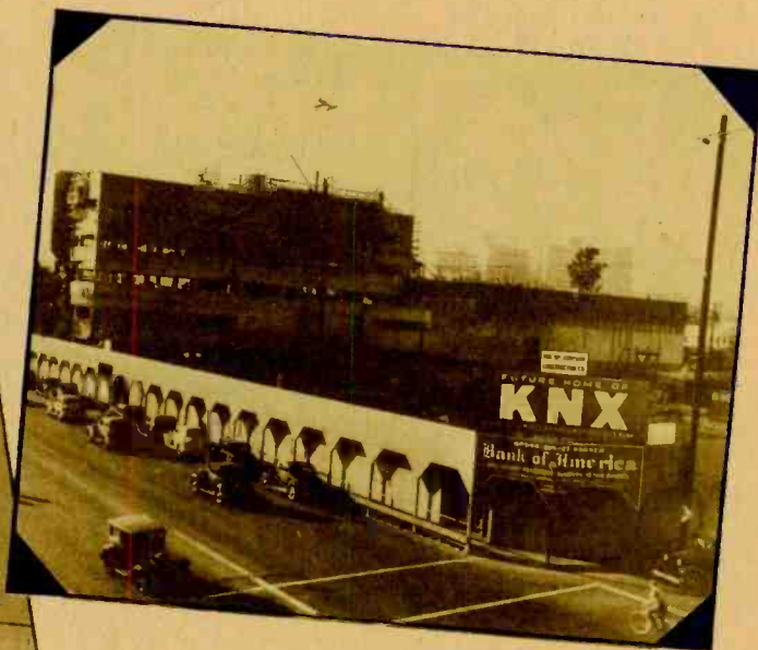
(Left) Laying the cornerstone at Columbia Square; (right) the studios under construction c. 1937.
