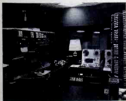
KSTP's Control Room.
