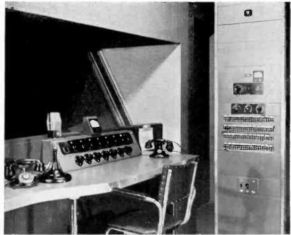
Cabinet type racks house the Western Electric 104A, 105A and 94C amplifiers with which each studio is equipped. The design of the control console permits, full, unobstructed view of the studio.
