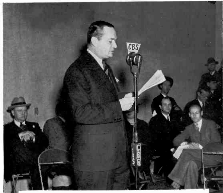
CBS reaches a milestone—lays a cornerstone. Vice-president Donald W. Thornburgh tells about it as ground is broken for Columbia's $2,000,000 studio and office building in Hollywood.
