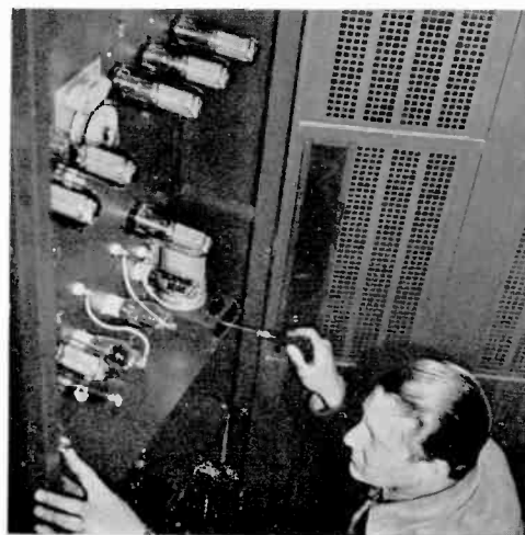
Engineer tuning the 702A oscillator. Left: The Western Electric 23A transmitter. Right: WCPO's vertical radiator, with Cincinnati's skyline in the background.
