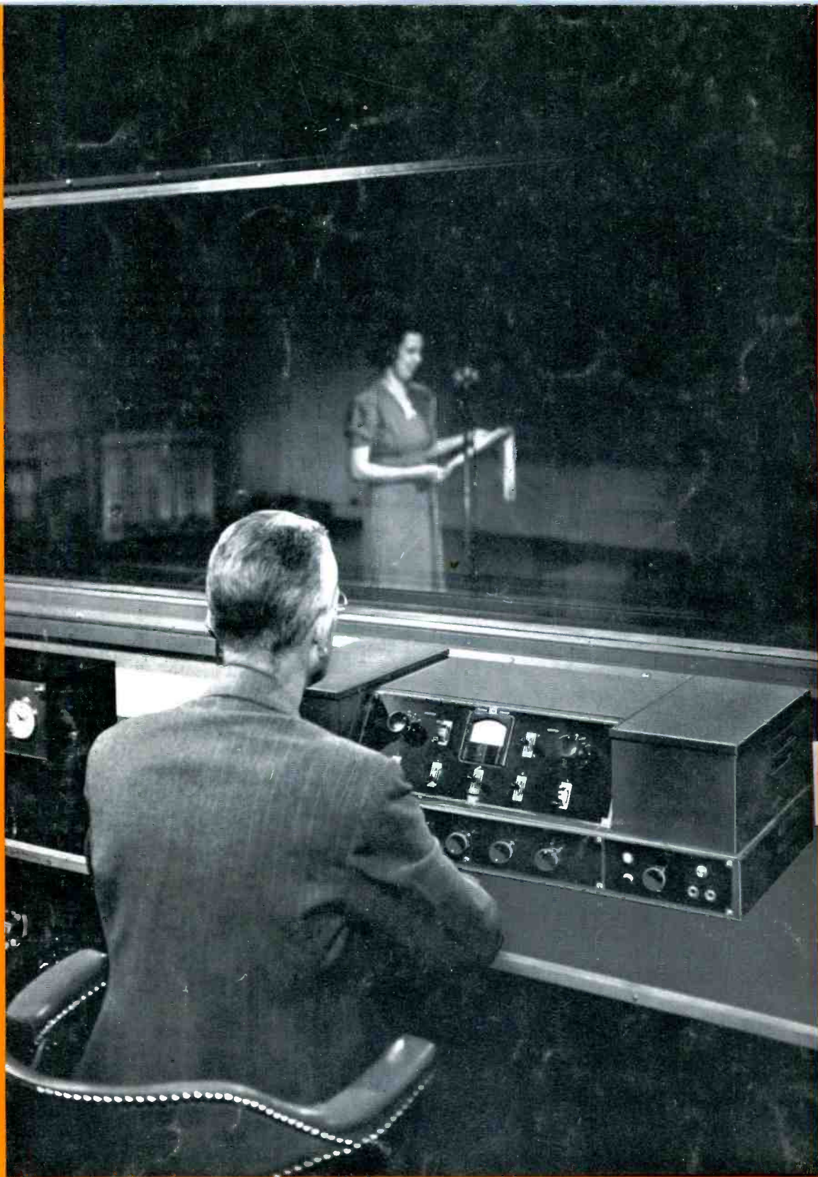
Western Electric 23B Studio Speech Input Equipment in a studio at CBS station WABC, New York, N. Y.
