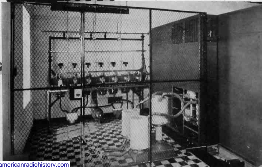
Rear view of transmitter showing rectifiers and water-cooling system for vacuum tubes.
