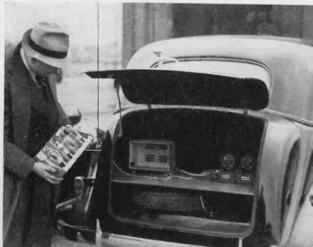
Right: Engineer Nolan S. Walker demonstrates how quickly mobile transmitters may be removed from metal cabinets for inspection.
