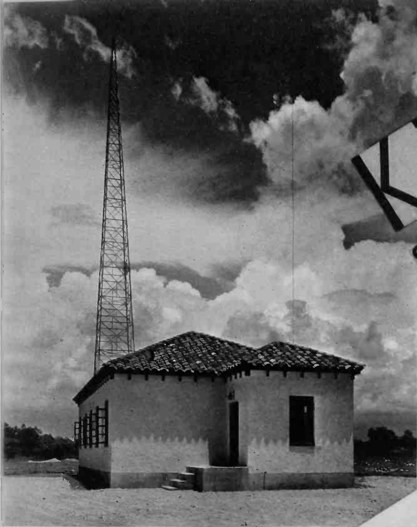
San Antonio's famous clouds form a colorful background for the new transmitting station and antenna.
