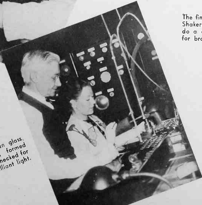
Checking air leakage. Just so much air—no more, no less—may filter through this silk-screen before it is accepted.
