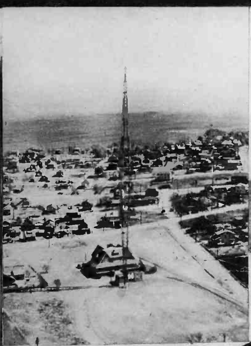
Four signals radiate from this mast
