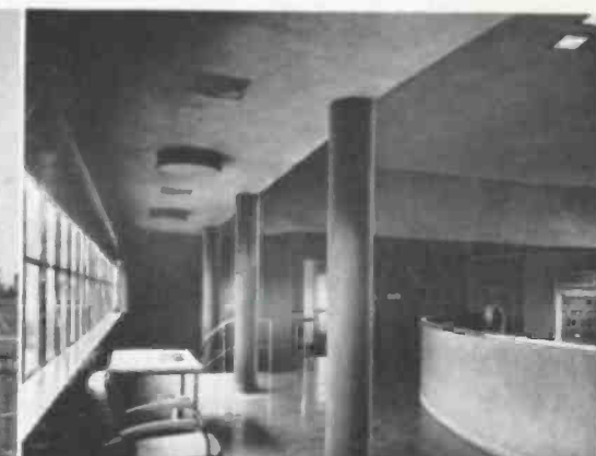
Lounge and control room observation
