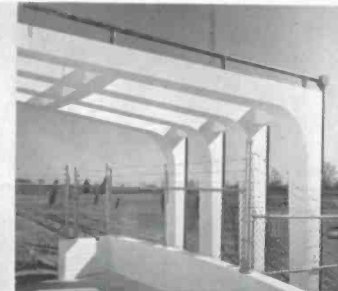
Arched columns support transmission lines.
