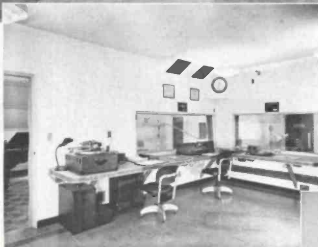
Above—Studio control area of transmitter and control room. Operator seated at the built-in desk in background has a view of both studios.
