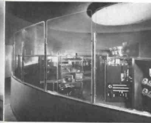
Rear of transmitter from observation area.
