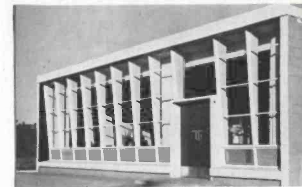
Glass front has overhang to control sunlight.
