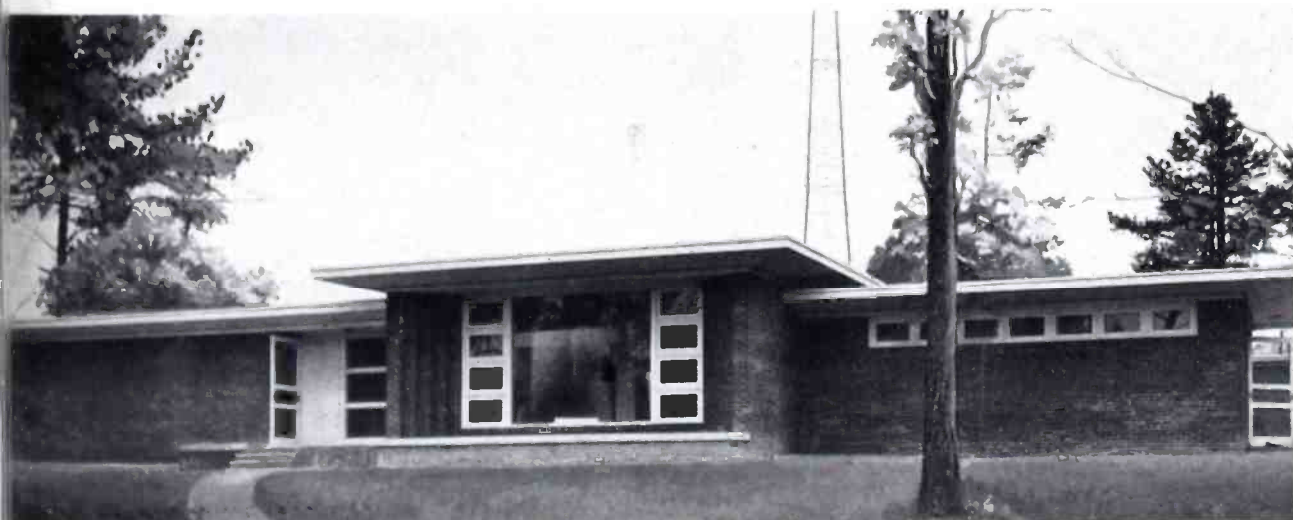
Sweeping modern exterior of new transmitter building for WDNC and WDNC-FM is expression of efficient planning which made it ideal dual AM-FM transmitter plant.
