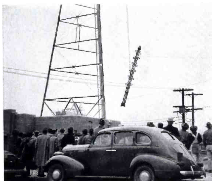
Six-bay Clover-Leaf antenna starts toward the top of the 450-foot tower erected in back of WFMY's modern studio-transmitter building.
