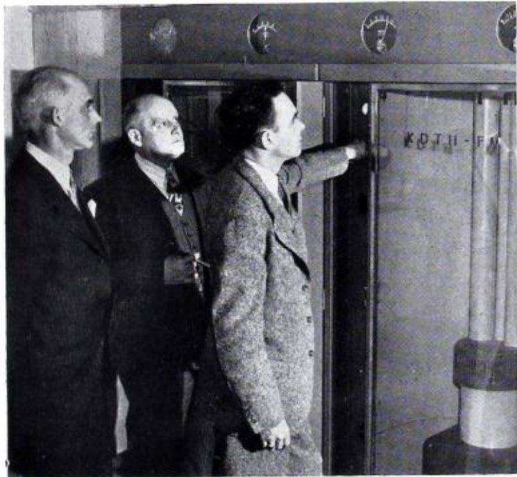
W. R. Emerson, KDTH and KDTH-FM engineer, and F. W. Woodward, President of the Telegraph-Herald Company, watch while R. M. Davidson of Western Electric throws switch to start KDTH-FM's 10 kw transmitter.
