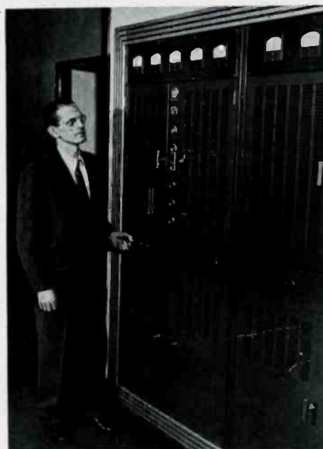
Chief Engineer C. F. Daugherty inspects the completed installation of new 50 kw transmitter.
