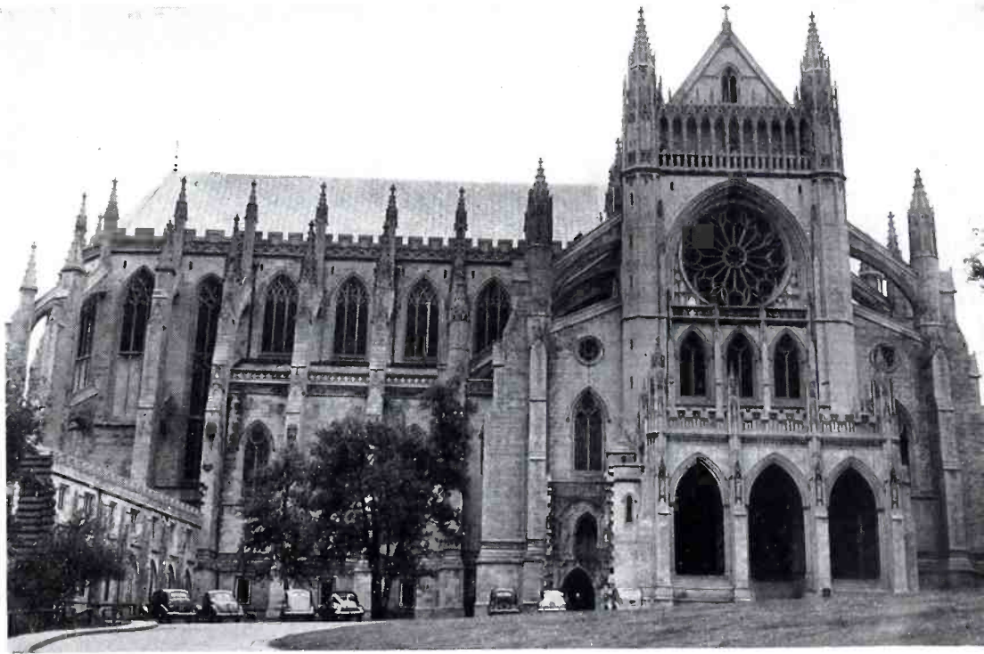
Another use of these loudspeakers is in finer reproduction of the services in great churches such as St. Albans Cathedral in Washington, D. C. Loudspeakers give a new quality realism and "presence".
