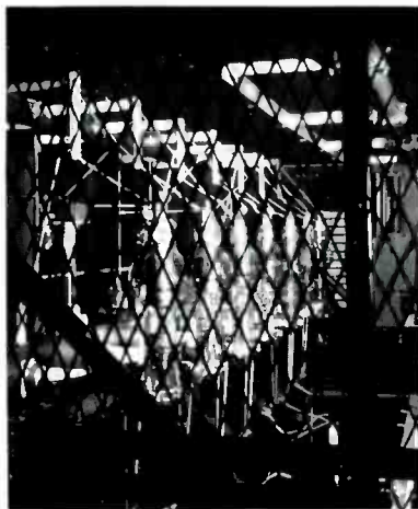
Row of seven mercury vapor rectifier tubes at KOMA.
