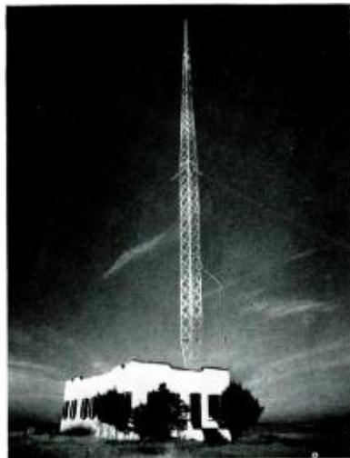
KOMA's old transmitter building with its 195-foot antenna. Building houses early 5 kw transmitter.
