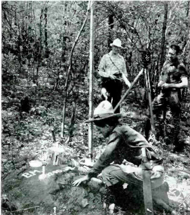
1. Preparation of site. Surveyors establish benchmark on rock at site of first relay station on Jackie Jones Mountain, 6 miles northwest of Haverstraw, N.Y.
