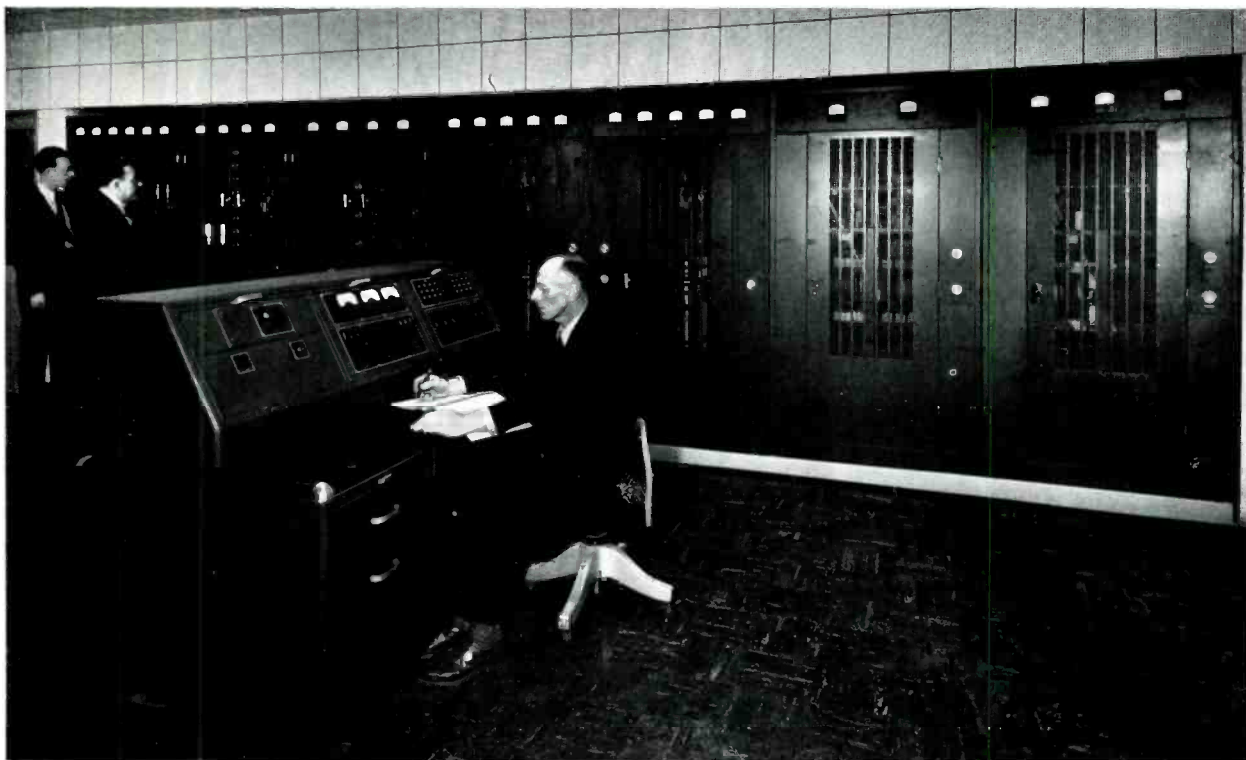
View of KOMA's new 50 kw Western Electric transmitter with KOMA's chief engineer M. W. "Tommy" Thomas seated at the Transmitter Control Desk. This equipment is housed in the brand new transmitter building shown on page 12. Standing are Western Electric Radio Engineers J. C. Herber (right) and K. K. White.
