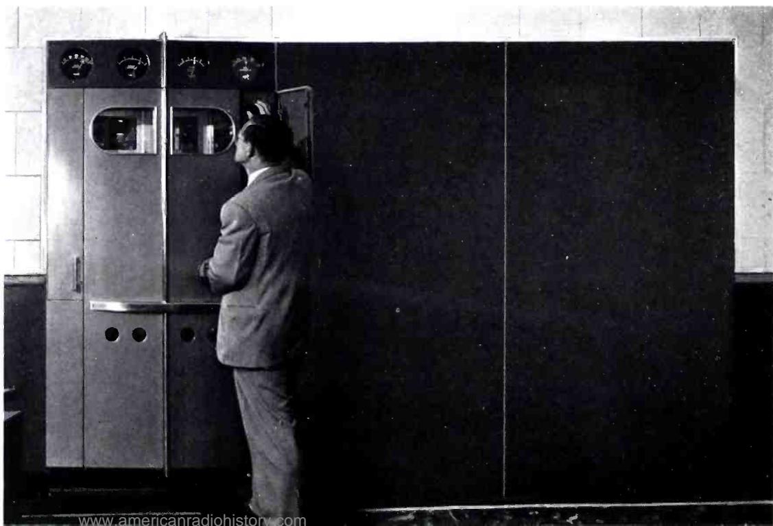
Paul Fuelling, chief engineer, checks the 1 kw Western Electric FM transmitter at WMGM. The blank area at the right will be filled by additional units which will give the station a power of 10 kw.
