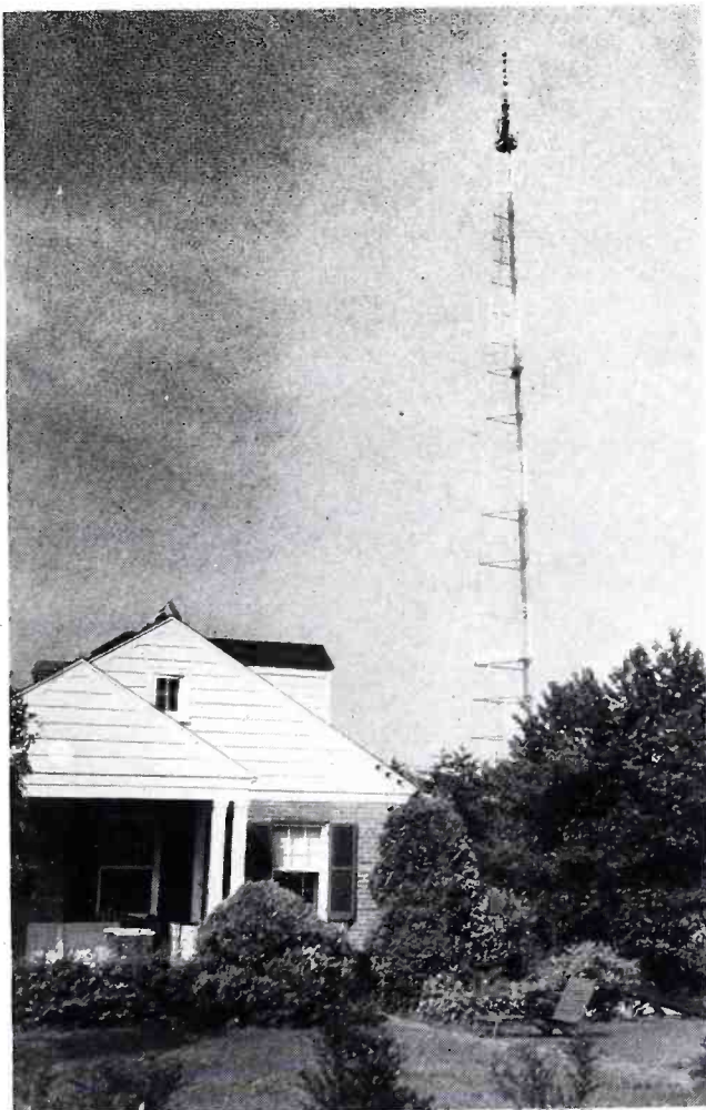
Silhouetted against the sky across the Potomac from Washington, D. C., is the 300-foot antenna tower of WINX-FM with its 4-element Western Electric Clover-Leaf Antenna.
