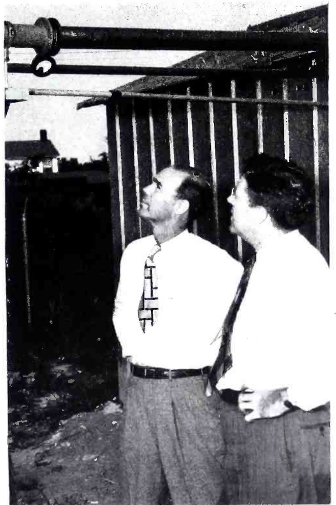
Engineer Cannon and John Aitkenhead, Western Electric broadcast field engineer, look over installation of coaxial type bridge developed by Bell Telephone Laboratories.
