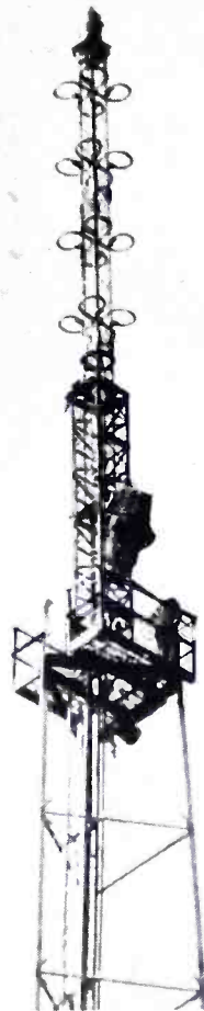
Close-up of a Clover-Leaf. This is the top of the antenna at left as seen through a telephoto lens.
