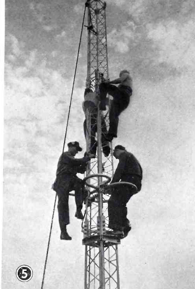
4. The second "A" section is in upright position about to be raised . . . 5. The second "A" section is erected and the splice bolts are being tightened at the same time the first clover-leaf is being assembled. Note that the gin pole is lashed to the first "A" section. The 20-foot length of 3-inch conductor has been assembled in the center of the tower. Steps are provided in one face of the tower
