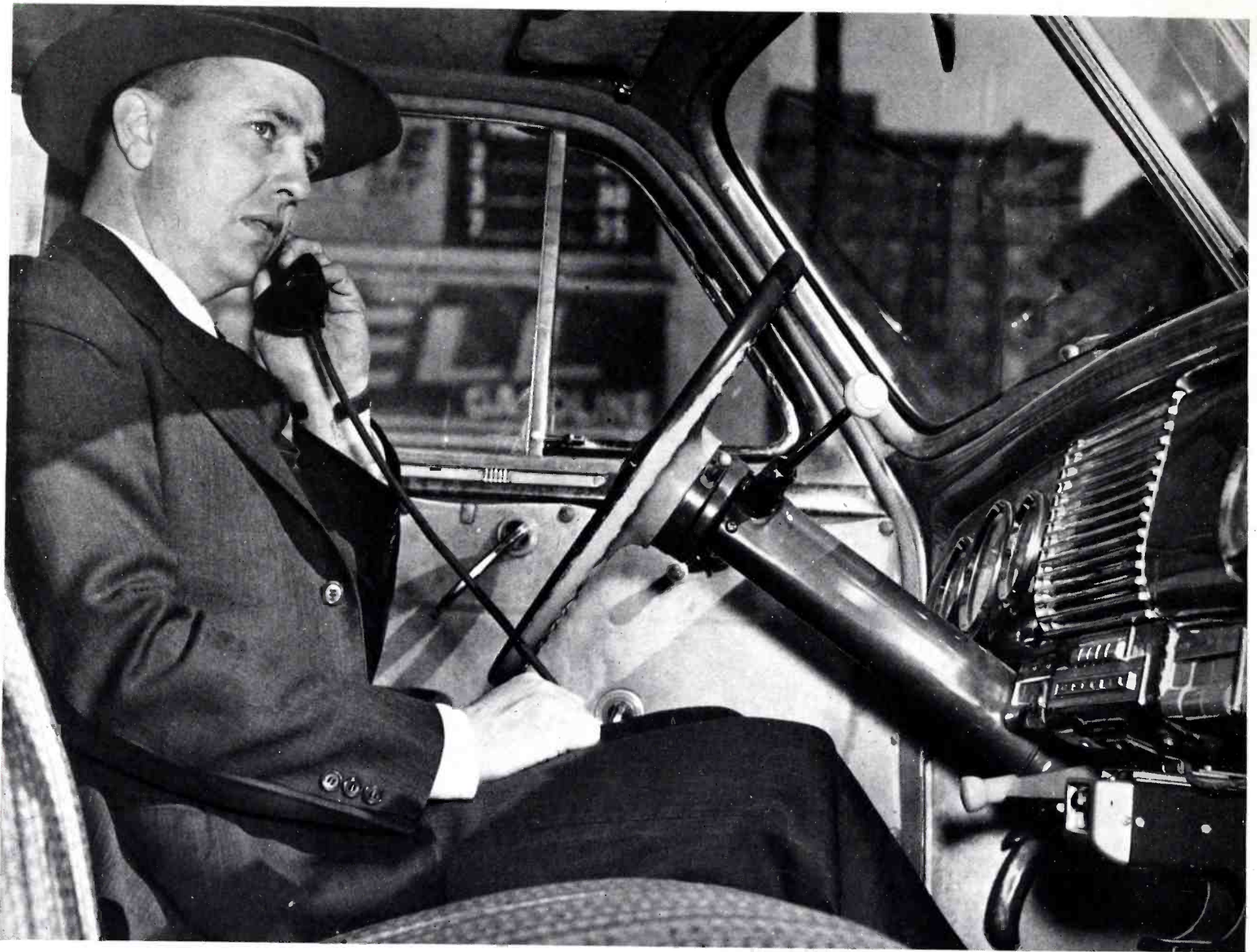
The only part of the mobile radio equipment visible to the vehicle operator is the 41A Control Unit. This is mounted conveniently beneath the instrument panel.
