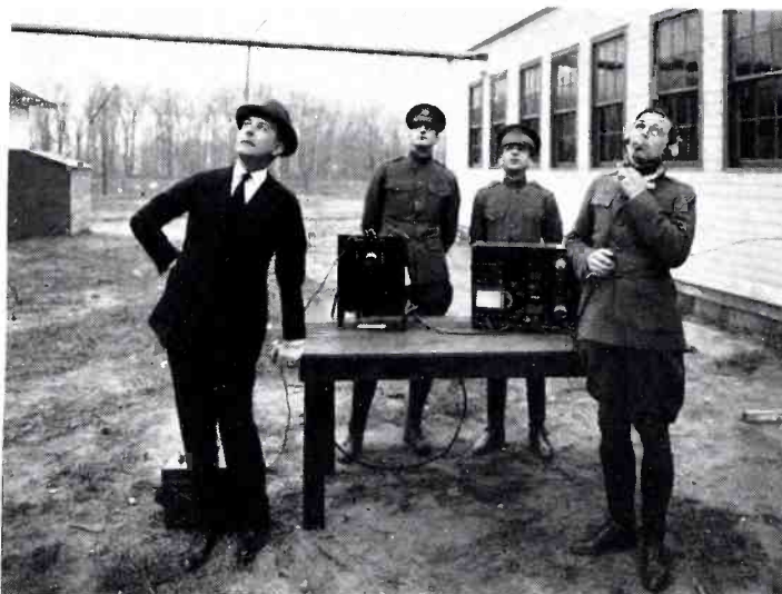
In August 1917 Western Electric engineers made the first radio telephone contact between the ground and a plane in flight. Above is the ground equipment used in the experiment. The demonstration was later repeated for President Wilson on White House lawn.
