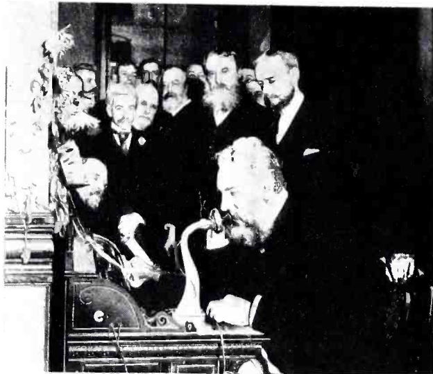
In 1892, Alexander Graham Bell, seventeen years after his historic invention, makes the telephone call which opens the first direct circuit between New York and Chicago. No repeaters were used. It was necessary to speak very loudly and clearly.
