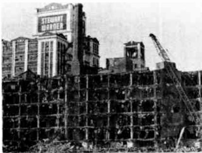
Partly-demolished Stewart-Warner plant under wrecker's ball in March, 1994.
