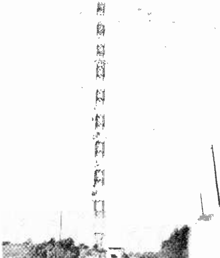
The 800 Foot Vertical transmitting antenna, NRS (T), Annapolis, Md. All wiring on the project was supervised by Electronics Division, PW Department personnel.
