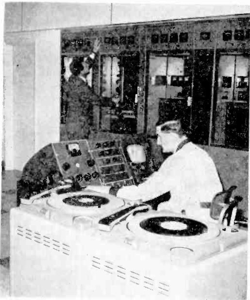
Fig. 5. CHCH-TV Audio and Video Transmitters and Transmitter Control.
