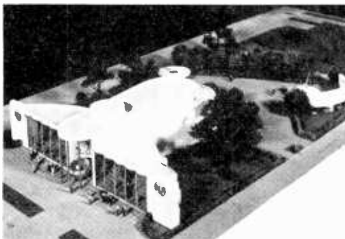
Model of R.C.A. exhibit building to be erected at the New York World's Fair 1939. It will be shaped like a Radio tube. Television programs will be featured.
