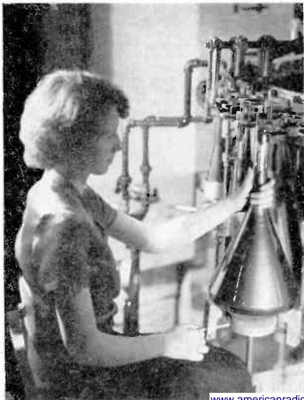
Fig. 8. Cementing base to tube.
