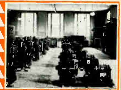
Above—Receiver, English and Australian circuits of the Yamachiche Beam Station. Below—Power Apparatus Room, showing incoming power control switchboard on right and main control switchboard on left, Drummondville Station
