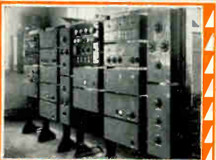
Above—Receiver, English and Australian circuits of the Yamachiche Beam Station. Below—Power Apparatus Room, showing incoming power control switchboard on right and main control switchboard on left, Drummondville Station
