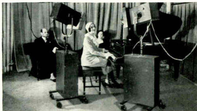
Courtesy Jenkins Television Corp. Pianist and singer before the Photo-Electric Cells of Television Station W2XCR and broadcasting sound station WGBS
