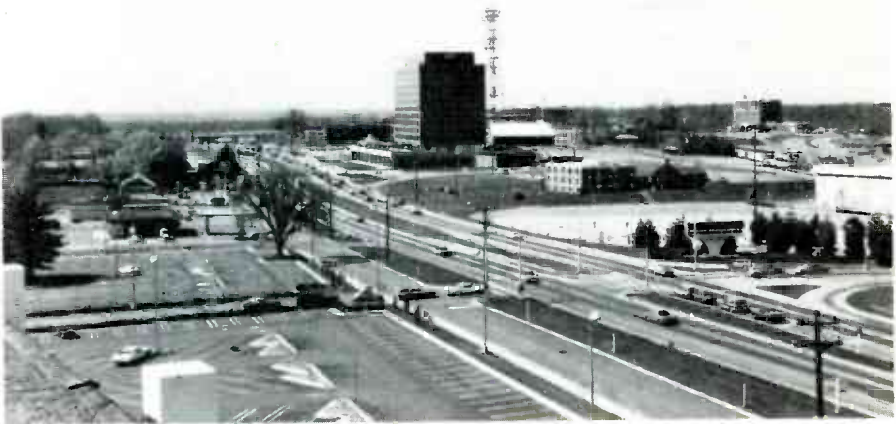
FIGURE 6. LOOKING BACK AT THE WR4ABR RECEIVER SITE FROM THE TRANSMITTER SITE.
