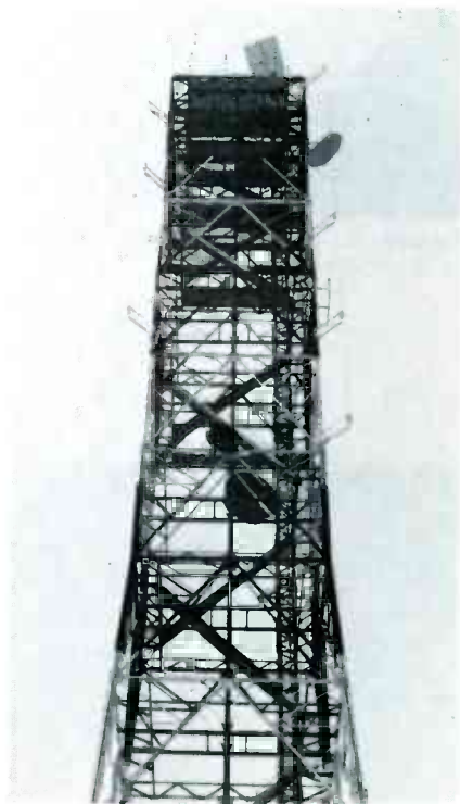
FIGURE 4. THE RECEIVER AND ANTENNA TOWER.
