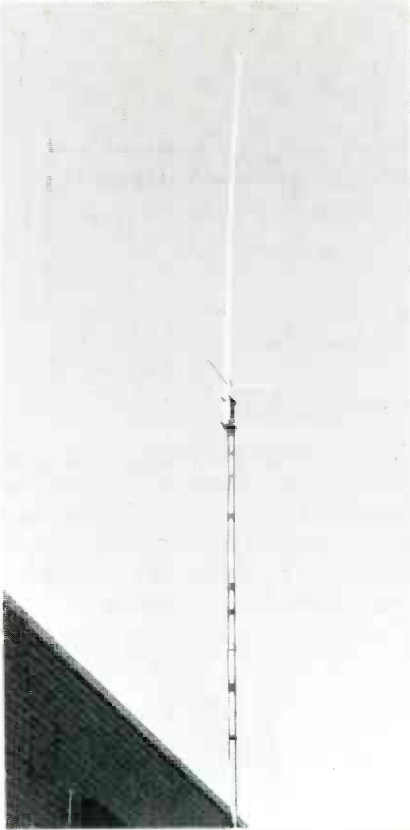
FIGURE 5. THE TWO-METER TRANSMITTER ANTENNA.
