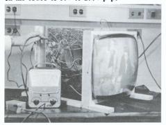
FIG. 7. Measuring peak-to-peak drive to CRT with special probe and Model 211 vtvm.
