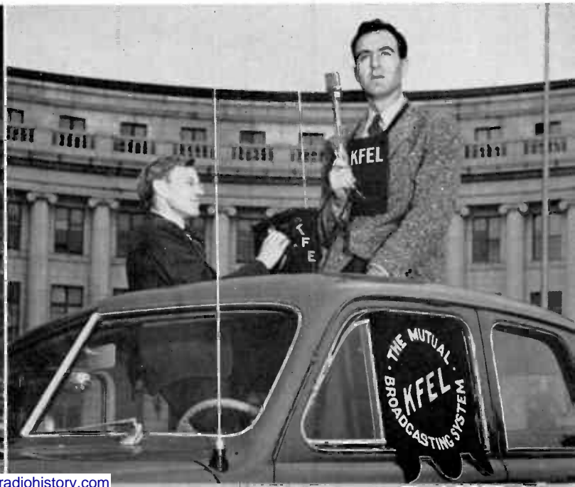
OBSERVATION CAR with sliding top and portable transmitter aids eye-witness broadcasts.
