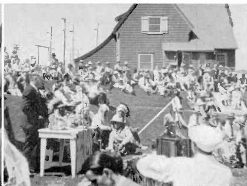
FLATHEAD INDIANS join celebration of completion of Kerr Dam on Flathead River in far west.
