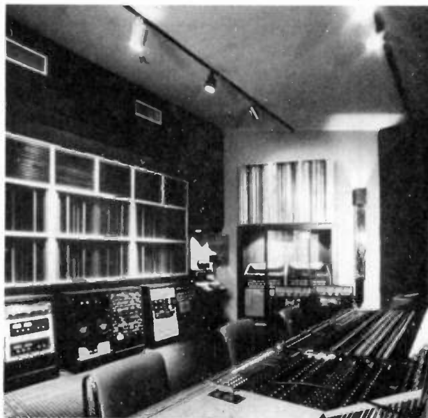
Figure 10. Rear view of the control room at Master Sound Astoria in the Kaufmann Astoria Film Studios, Astoria, New York, showing rear and side RPG clusters. Acoustical consultant Charles Billelo Associates.
