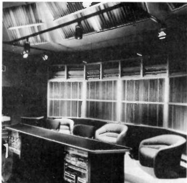
Figure 9. Rear view of the control room at Tele-Image, Dallas, TX showing the upper and lower RPG clusters. Acoustical consultant Russell Berger, Joiner-Rose Group.
