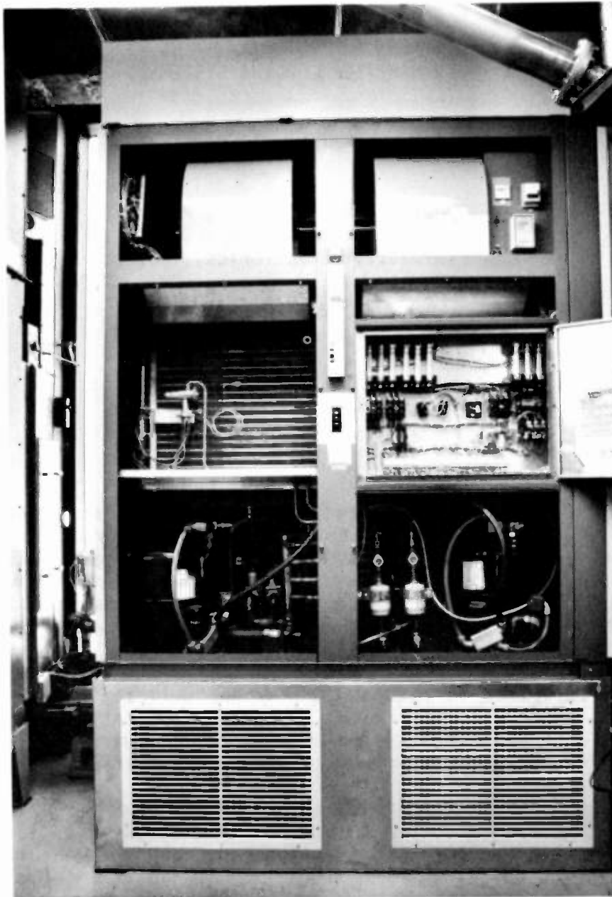
PHOTO - 2 This picture shows the front view of the package cooling unit with service covers removed. The air flow is downward; a base with grills direct the air flow along the floor. The ctangular box on the top houses the economy cooling coil, and frame for the air intake filters. The unit is 5 ft. wide by 8.5 ft. high.
